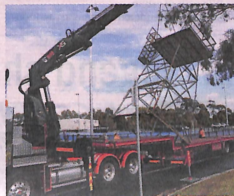
The Plunkett's crane truck lifts its towering cargo. 233809
