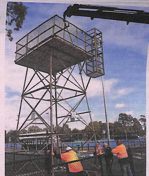
The ladder tower is set in place near the Olive Road running track. 233809
