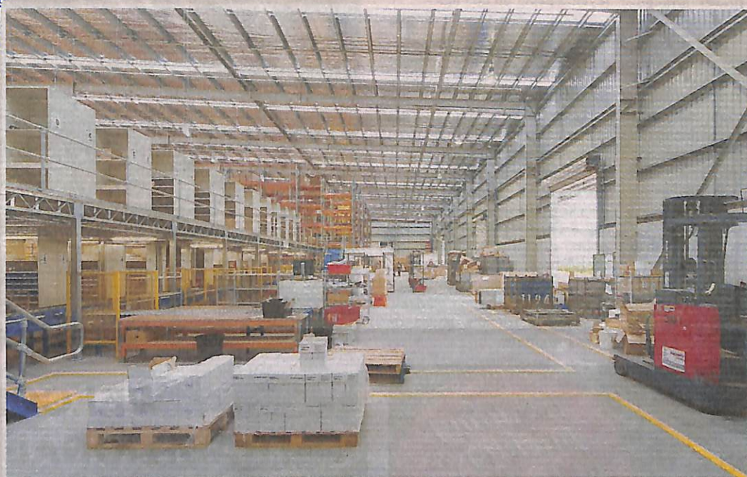
The new warehouse space.
