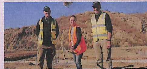
Ward Petherbridge, Dandenong MP Gabrielle Williams and Geoff Petherbridge turn the first sod of the new facility. 191904 Picture: STEWART CHAMBERS
