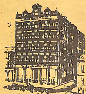
THE original Rocke Tompsitt Warehouse in Flinders St.
