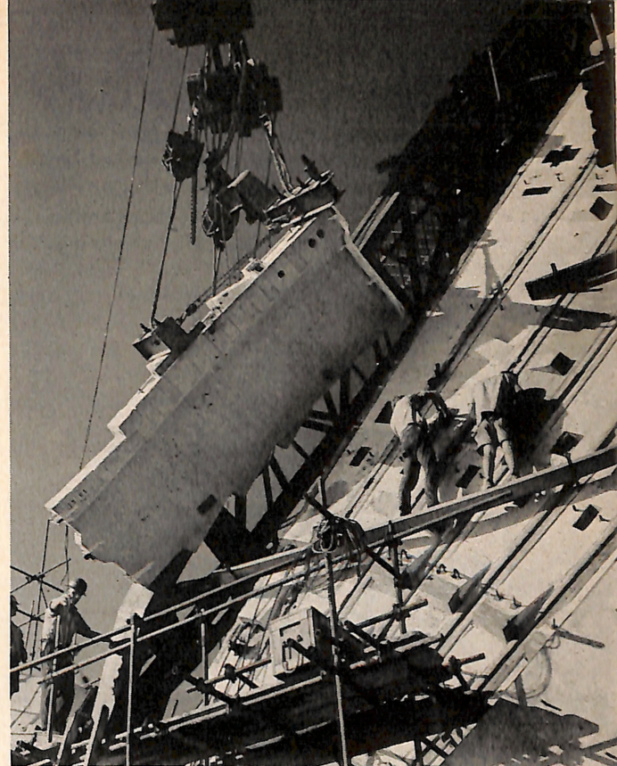
Builders have evolved a telescopic erection arch (black diagonal girders) which is used to place weighty concrete rib elements in precise position. These are prefabricated in workshop.
