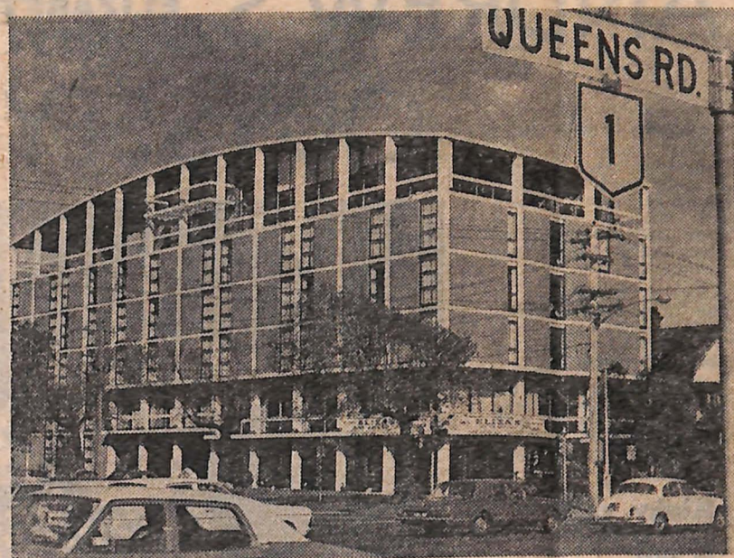
JOHN BATMAN MOTOR INN, Queen's Rd., was one of the first motels to get away from dull, box-like lines. The curved ceiling houses a two-level penthouse apartment.
