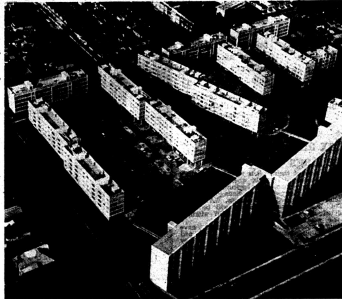
Flat-building is booming—even in outer suburbs
