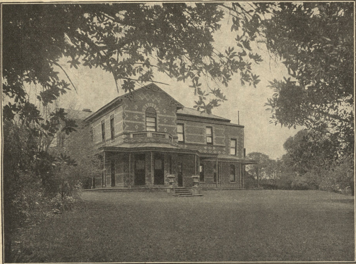
THE BOARDERS' HOUSE.
