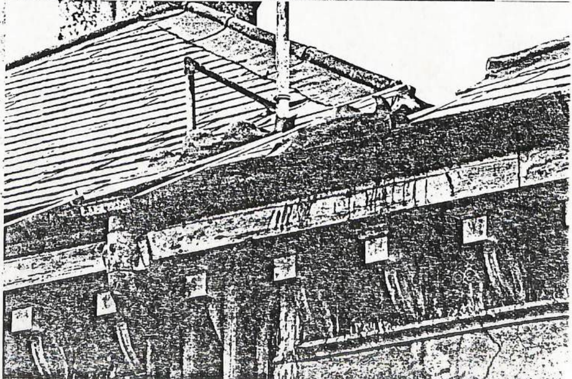
Downpipe and cornice at upper roof north side.
