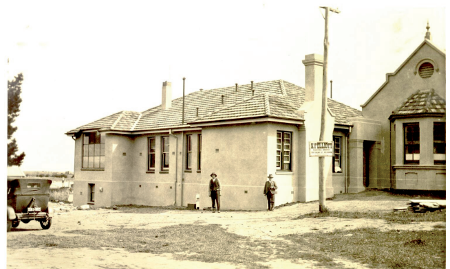
Photograph of the 1934 hospital building works
