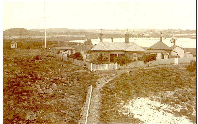
Lighthouse Keepers' cottages
