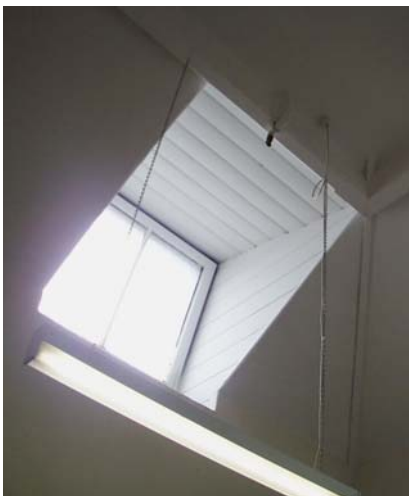
5. Timber-lined skylight in stairwell
