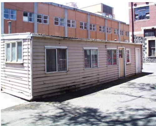
5. Store, south-west view
