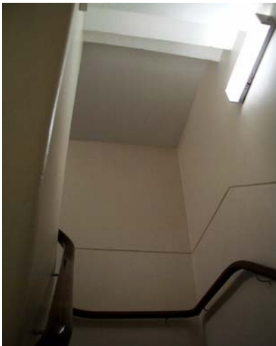
5. Stairwell to first floor
