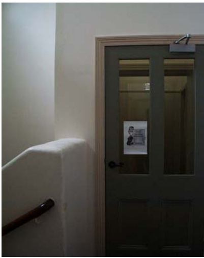
3. Non-original entry to stairwell
