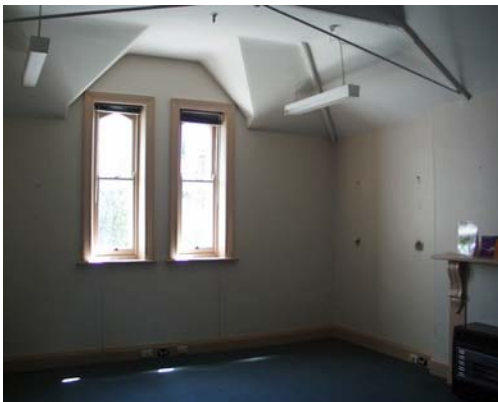
3. Typical corner office, second floor
