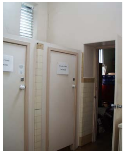
6. Female toilets and former shower area
