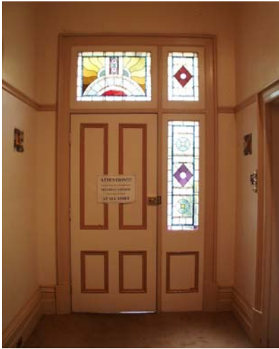
1. Non-original entry to north wing
