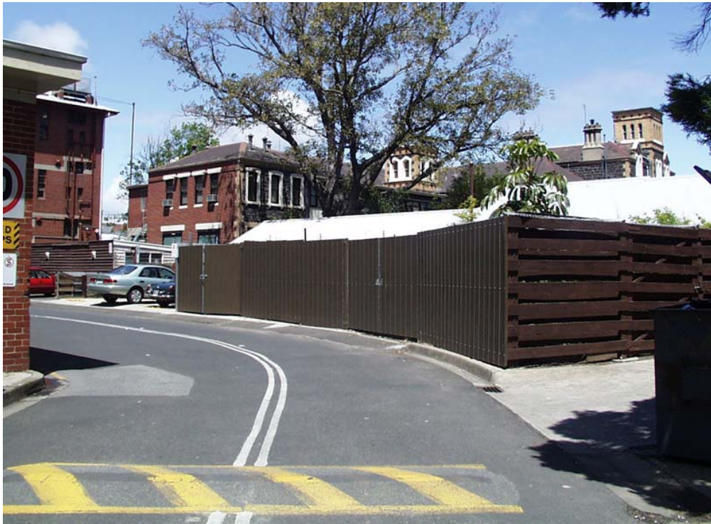
Figure 14 View of the Institute building (in the background) from the Alfred Hospital site to the north
