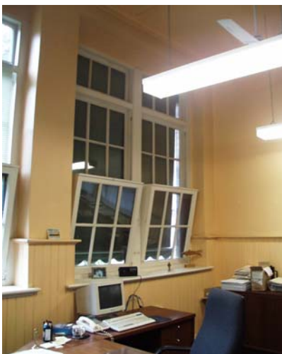
5. Office, north-west corner
