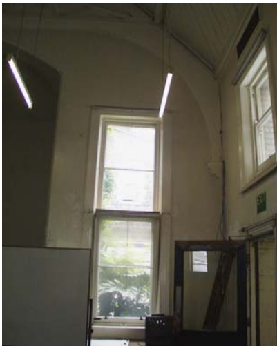
5. Window detail east wall
