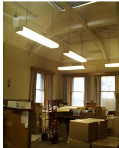
4. Store room G.27, north wing
