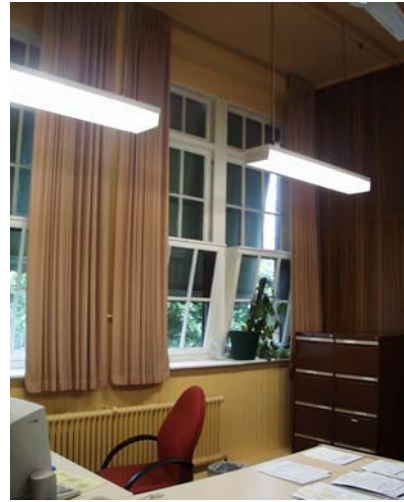
2. 1932 west wall window and dado
