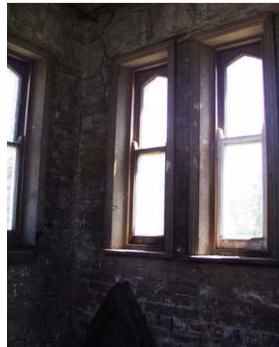
3. Central turret walls
