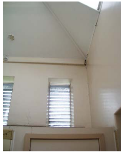
4. Raked ceiling in toilet
