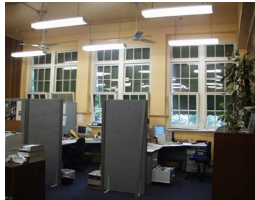
4. Pairs of windows, west wall
