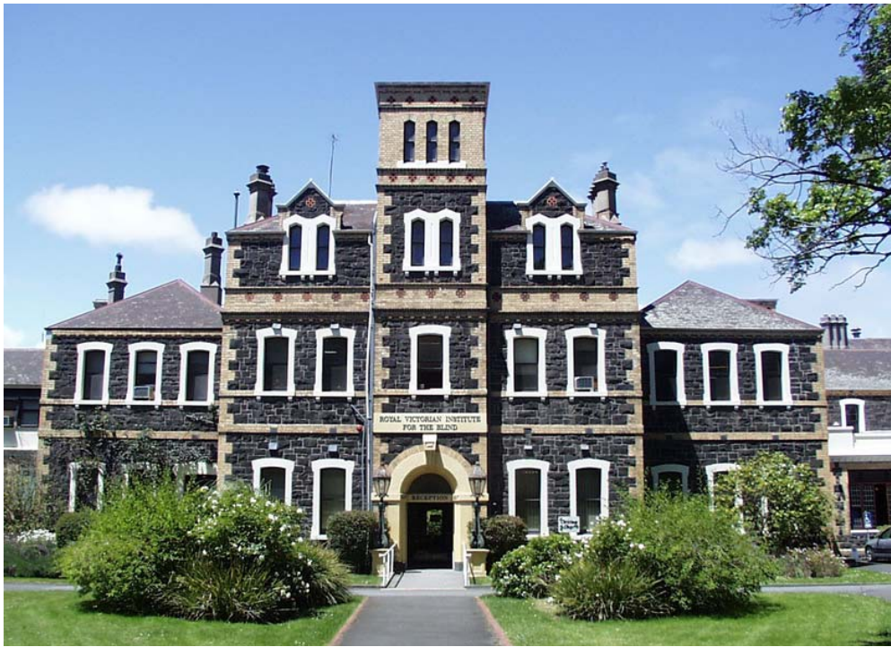
Figure 19 RVIB west façade facing St Kilda Road
