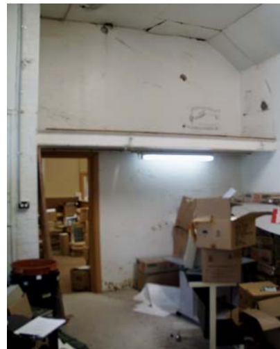
6. Storage mezzanine to G.31
