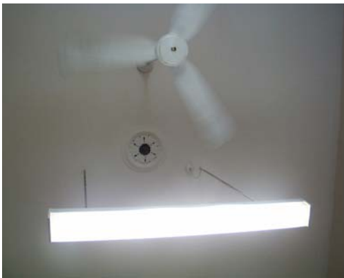
3. Ceiling ventilation rose in office
