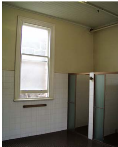
6. Non-original finishes to female bathroom
