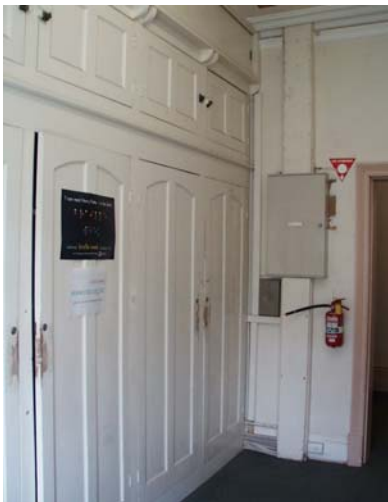
5. Detail of timber corridor joinery
