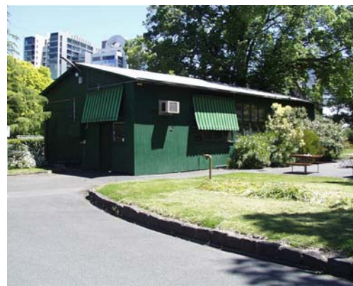
6. Former gymnasium, north-east view
