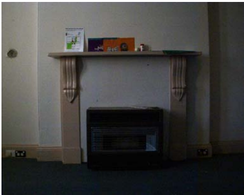
3. Typical fireplace, corner office
