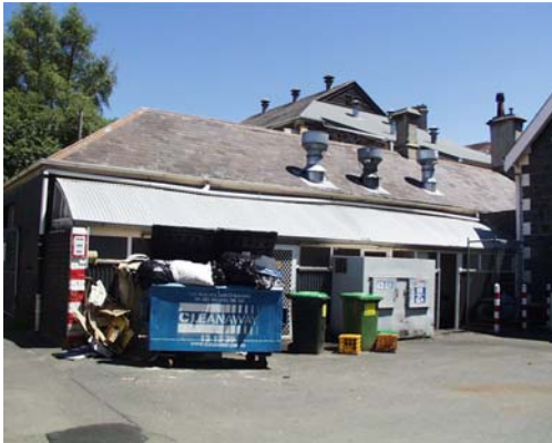
3. South wing rear elevation
