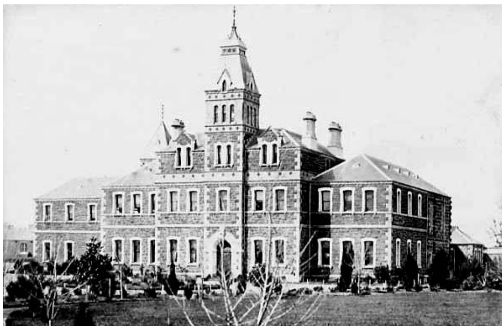
Figure 5 View of the RVIB building from the south-east c.1870 Source: State Library of Victoria Pictoria Collection
