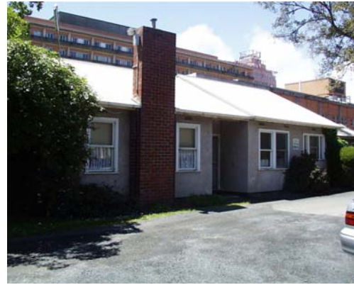
4. Myer House, south-west view
