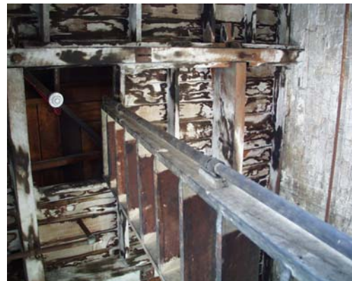
4. Access ladder to non-extant roof turret
