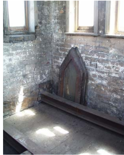
2. Central turret timber floor
