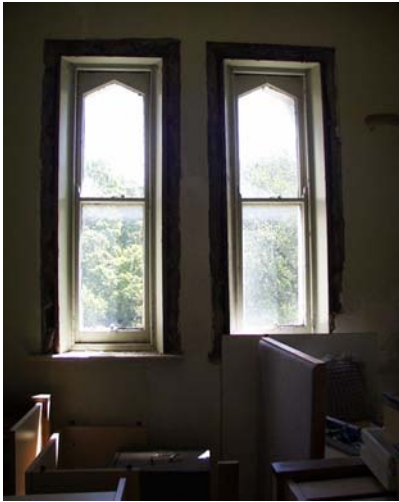
1. Central store room, second floor
