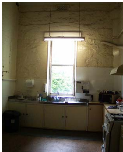
4. Kitchen north wall joinery
