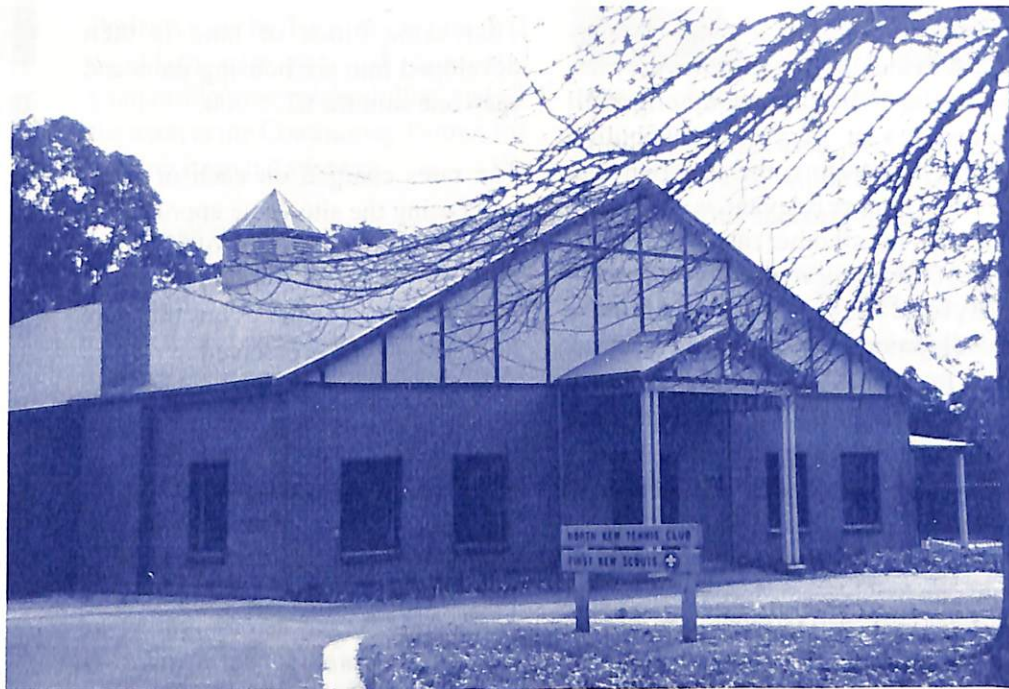
The new Tennis Club and Scout Hall Facilities.
