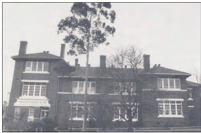
East Kew School No. 3161 in Kitchener Street.
