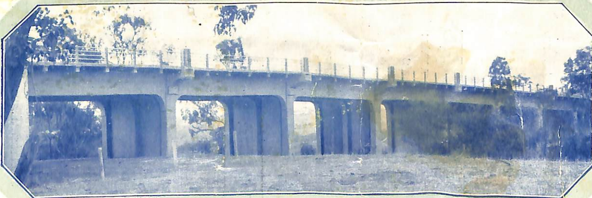
The new Burke Road Bridge that carries the great inter-suburban traffic.
