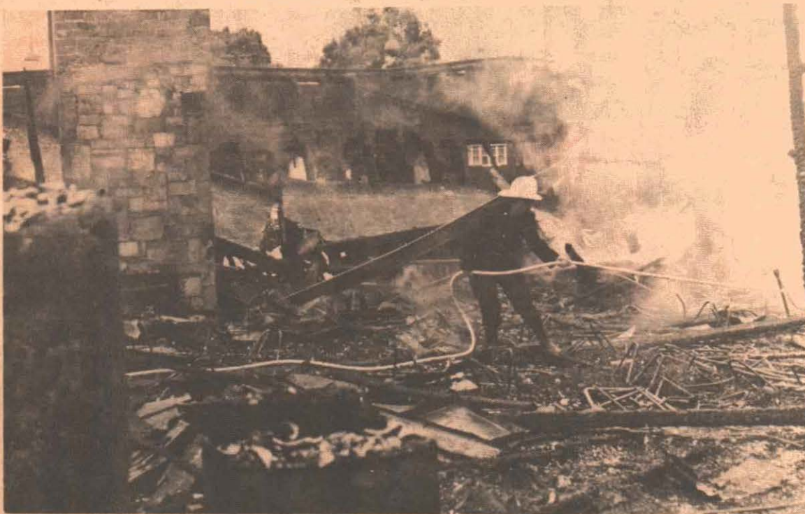
Fire destroyed Caulfield Park Bowling Club on Sunday November 20 at 5 a.m. The fire occurred just two months after the Conservatory, also located in Caulfield Park, was destroyed. Spokesman for the bowling club, John McDougall said "We lost everything, all trophies, honours boards and records. Fortunately I had the first six minute books at home, I was working on our club's history, and they are all that remains." Photograph by Bruce Dinan shows firemen at work amongst the rubble.
