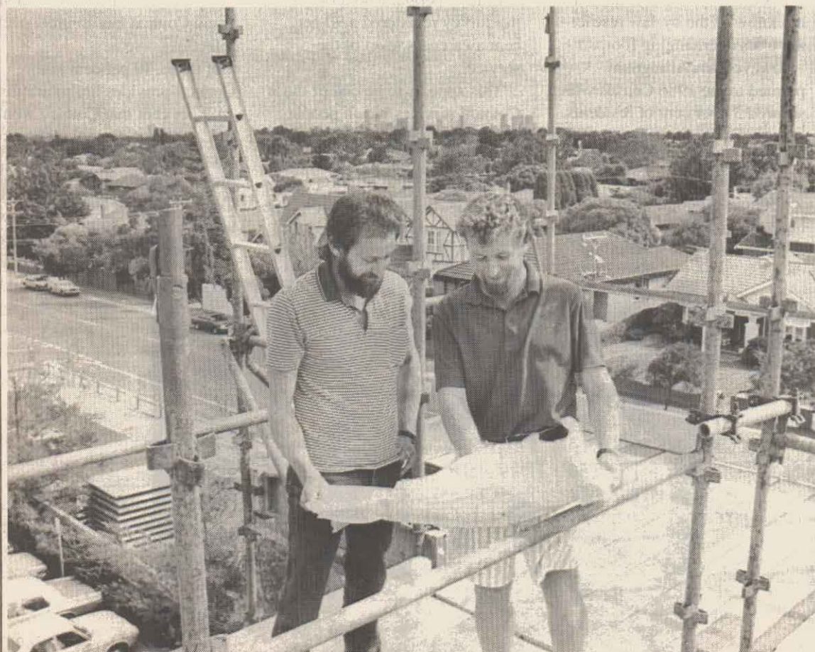
● Council building inspector Keith Franklyn (right) checks progress on City Hall extensions with foreman Doug Fullager.
