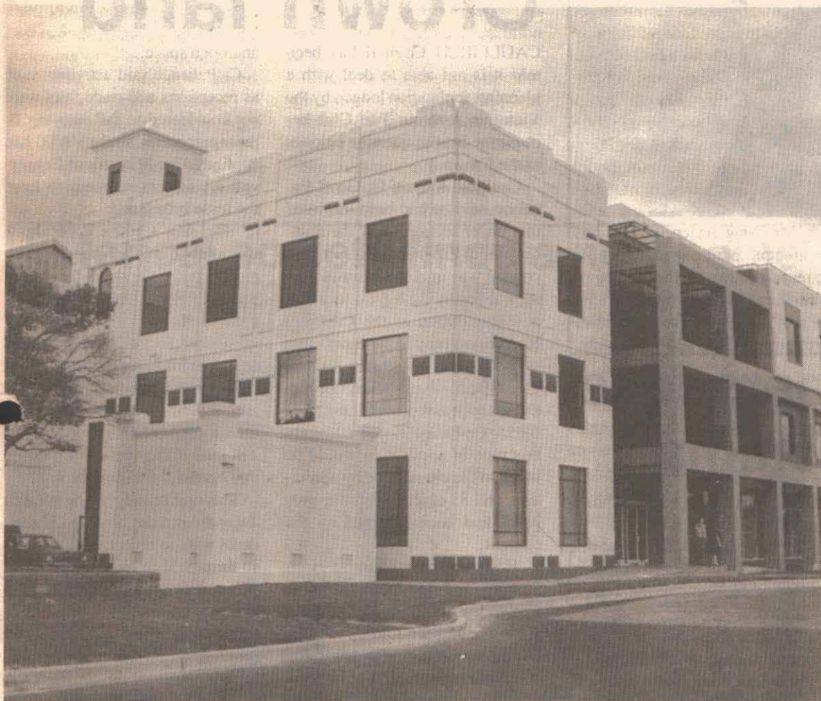
Above: After two years in the making, the extensions to Caulfield City Hall are now open.
