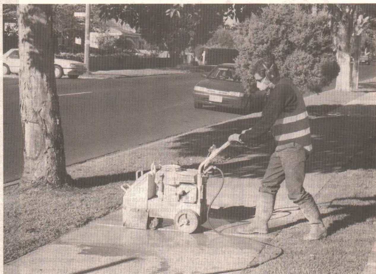
Grinder operator Tony Sammut smooths out a section of pavement in Neerim Road.
