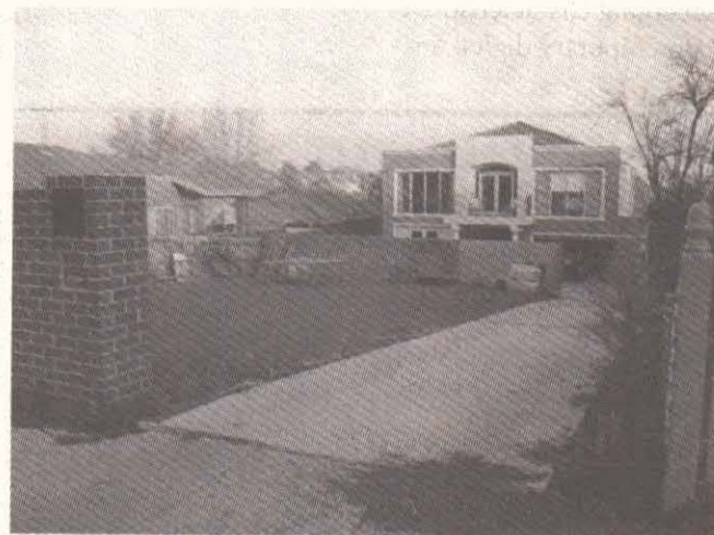
11 Ludbrook Avenue—house built at rear of property with dividing brick wall in front of it; second brick wall has been built at the front of property which allows for second driveway, entrance gate and letterbox.
