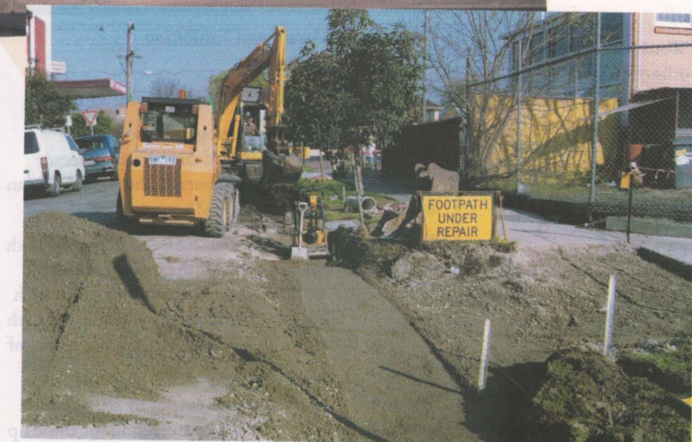
Catch up renewal works on footpaths and roads will continue throughout the City.
