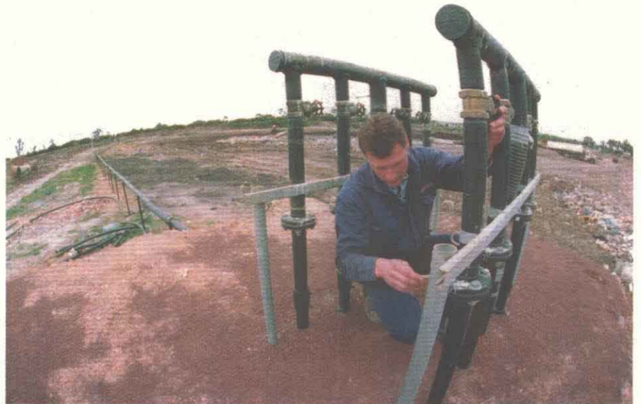
Site manager Damien Edmonds checks a gas extraction manifold at Clayton Landfill.
