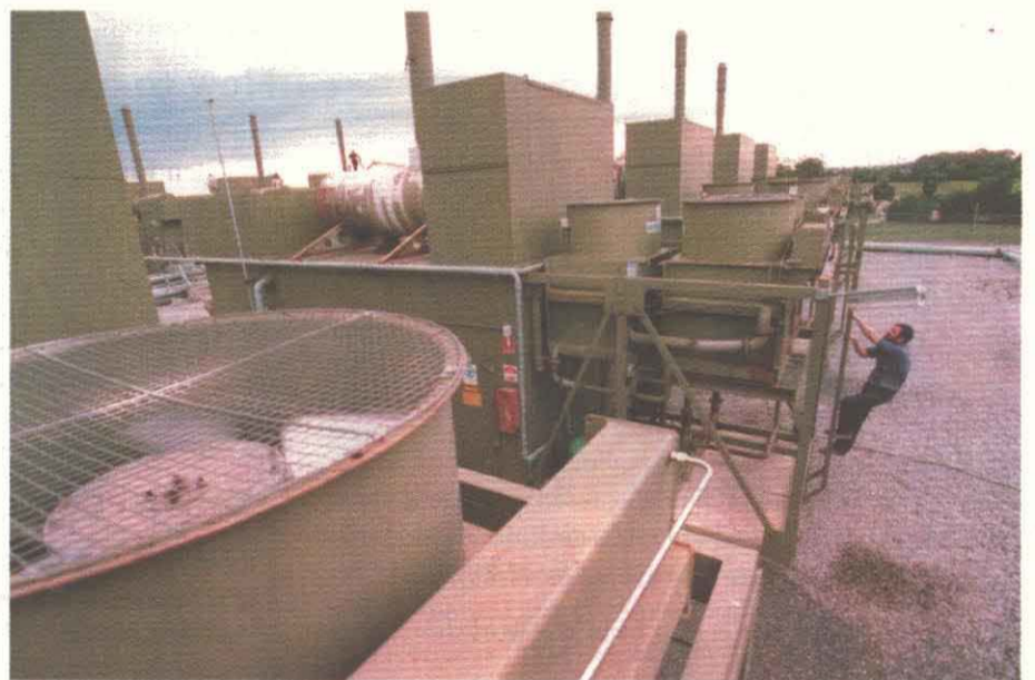
The huge turbines—each one capable of generating 1 million watts of electricity from methane. Photos: Bernie Bickerton.
