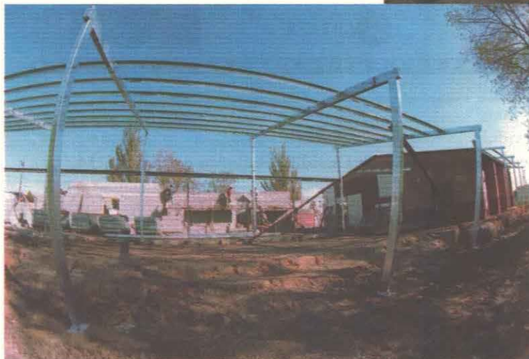
During: Construction of the pavilion also from the eastern end, showing the old hall.
