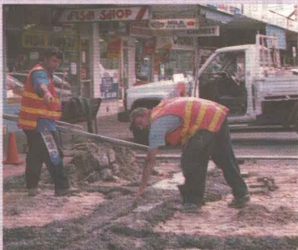
Workers install kerb extensions at the corner of Parkmore Road and Mackie Road as part of the Mackie Road shopping centre upgrade.
