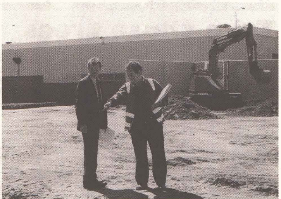
Manager Corporate Assets Tim Frederico (left) and GlenWorks staff member Roger Dunn discuss the finishing touches to the new depot yard.
