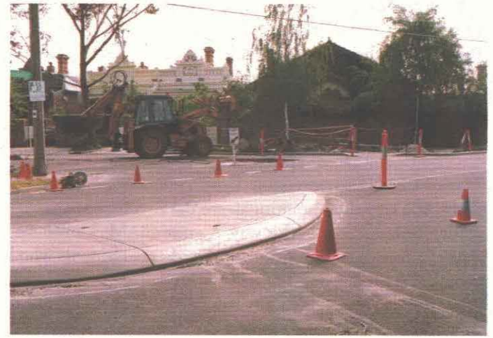
A new traffic island and right turn lane makes Kambrook and Normanby Roads, Caulfield North a safer intersection.
