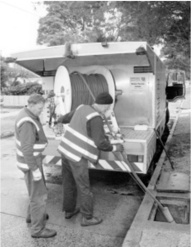
Council has upgraded its drain jet truck-an effective and efficient way to clear drains from tree roots. Photo: Maureen Bathgate.
