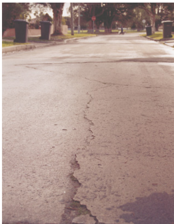
The ageing concrete road in Moira Avenue, Carnegie will be reconstructed to preserve its heritage qualities.
