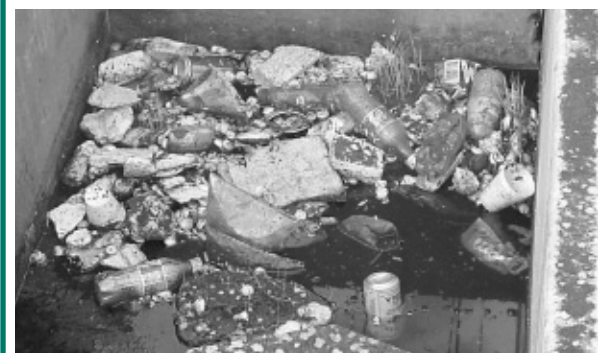
All this rubbish would have ended up in local waterways were it not for Council's new litter trap in Mitchell Street, Bentleigh.
