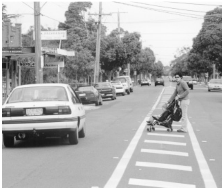
A newly installed chevron median provides a safe place for pedestrians to stop as they cross busy Booran Road near the shopping centre precinct. Photo: Bernie Bickerton
