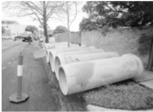
(inset) Council installed 240 metres of drainage pipe and new stormwater pits in the vicinity of Elizabeth and Sinclair streets.
