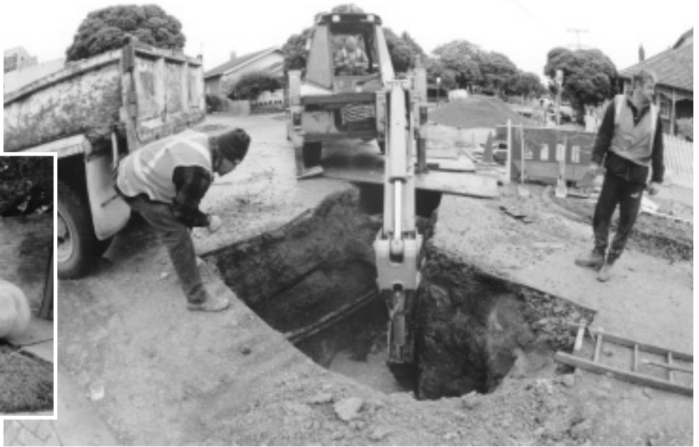
Recent drainage work in Elsternwick will greatly assist in the disposal of stormwater run-off in the area around Elizabeth and Sinclair streets. Photos: Bernie Bickerton.
