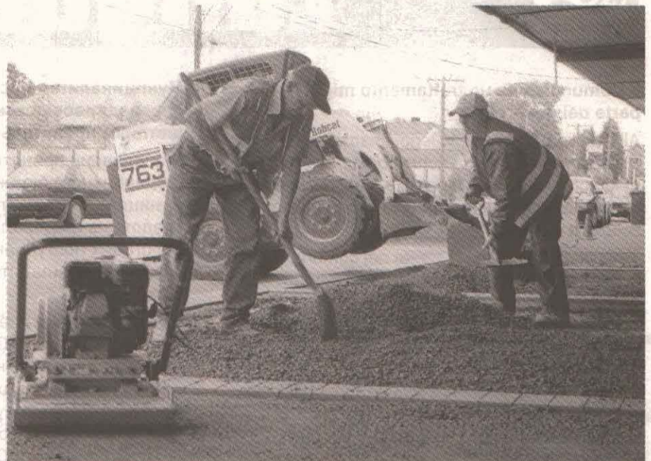
New paving, street trees and lighting is installed to revitalise McKinnon Shopping Centre. Photo: Myrine Hawksworth.
