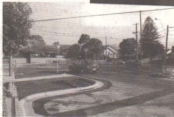
Roundabout installation almost complete at the corner of Kambrook Road and Station Street, Caulfield North.
