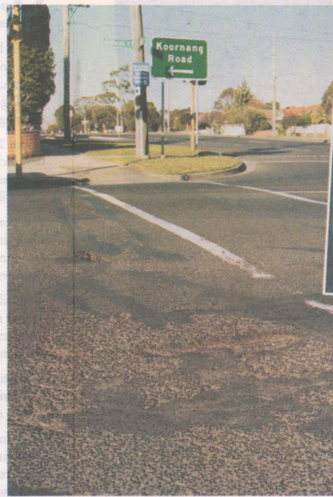
"Aging infrastructure" — cracking asphalt and damaged kerb and channel — a major focus of the budget.
