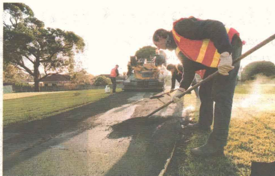
GlenWorks staff get an early start on bike path construction in Bailey Reserve. Photo: Bernie Bickerton.
