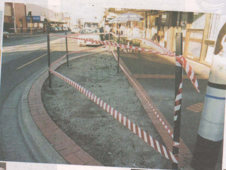
"Appearance of public areas" was named as a priority in the Community Satisfaction Survey — Glen Huntly shopping centre works.
