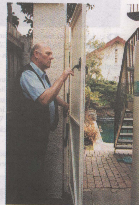
Building inspector Mervyn Mumford checks the installation of a self-closing device on a pool gate in Caulfield.
