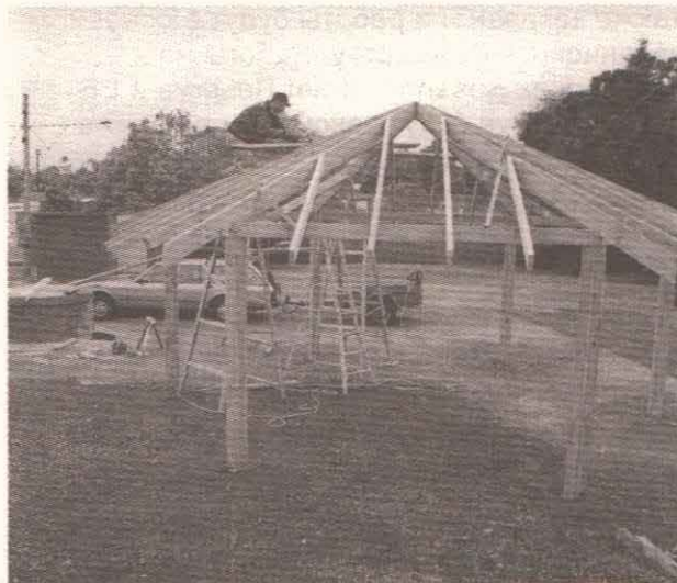
Marlborough Street Reserve upgrade is well underway as the new pergola is erected.
