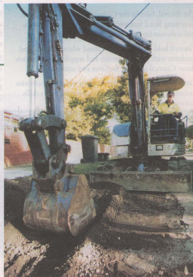
Workers prepare to install new drainage in Malane Street, Ormond. Photo: Bernie Bickerton.
