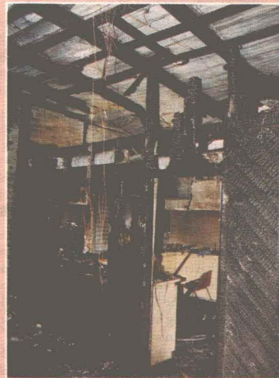
The pavilion suffered extensive structural damage in the blaze.
