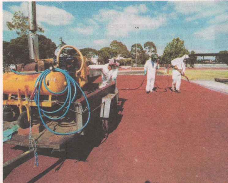
The new synthetic surface gets sprayed onto the athletics track at Duncan Mackinnon Reserve. Photo: Bernie Bickerton.
