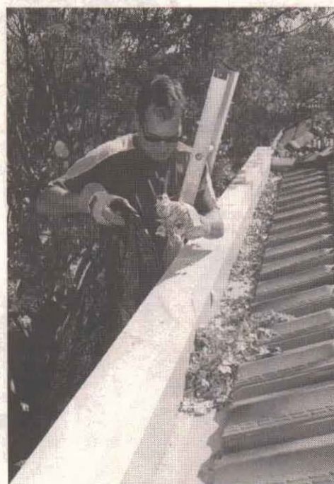
Murrumbidgee resident Jason Close cleans out the roof gutters on his home to ensure fallen leaves don't block the City's drainage system. Photo: Bernie Bickerton.
