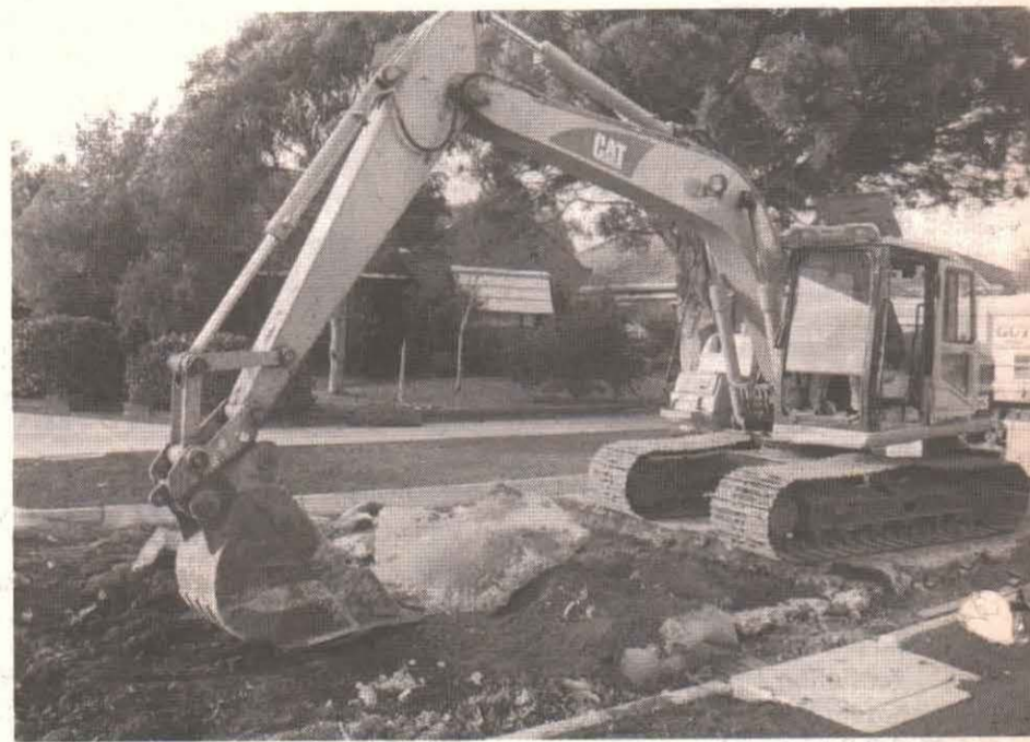
Old, damaged concrete pavement in Moira Avenue is removed to make way for the new road surface. Photo: Anne Stafford.
