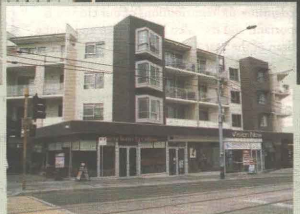
The Elsternwick Hub (right) is a good example of a residential development above shops in Glen Eira.
