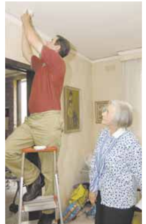
Property maintenance officer Peter replaces a smoke detector for Hania.
