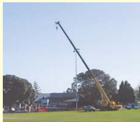
The latest technology in sportsground lighting has been installed at three of the four sportsgrounds located in Princes Park. Photo: Tracy Cassidy.
