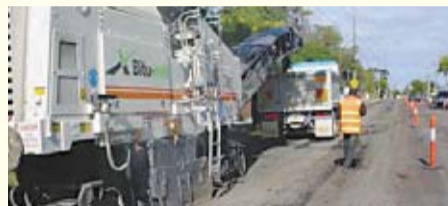
Road resurfacing along Kooyong Road between Glen Eira Road and Glenhuntly Road, Caulfield.
