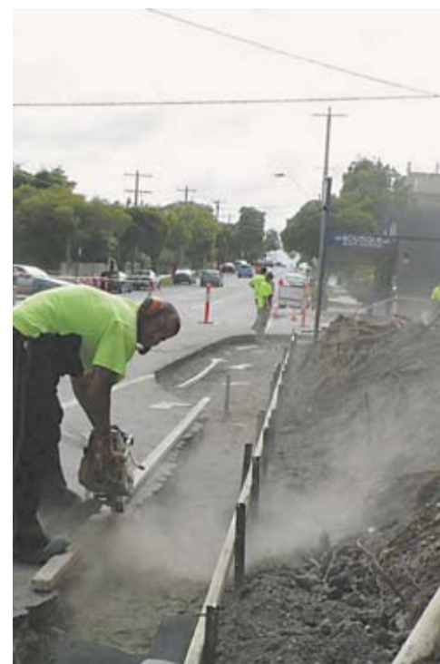
Works at the intersection of Gardenvale and Kooyong Roads, Gardenvale. Photo: Glen Eira City Council Capital Works Unit.
