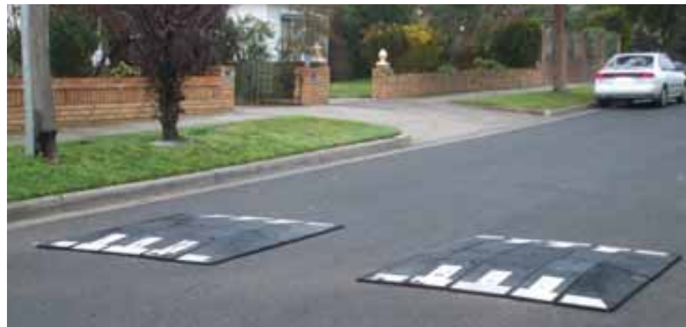
Recycled rubber has been used for speed cushions on Bellevue Road, Bentleigh East.
