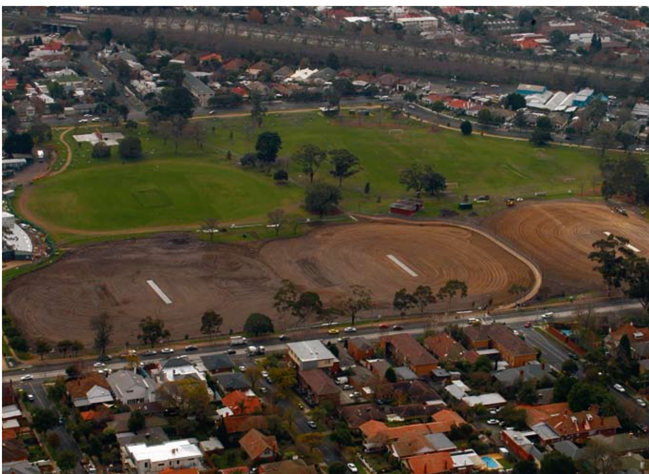
Resurfacing works at Caulfield Park.
