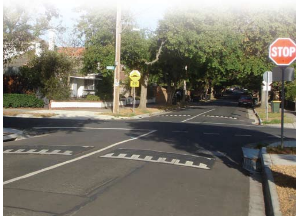
Speed cushions at Ludbrook Avenue and Lucas Street, Caulfield South.
