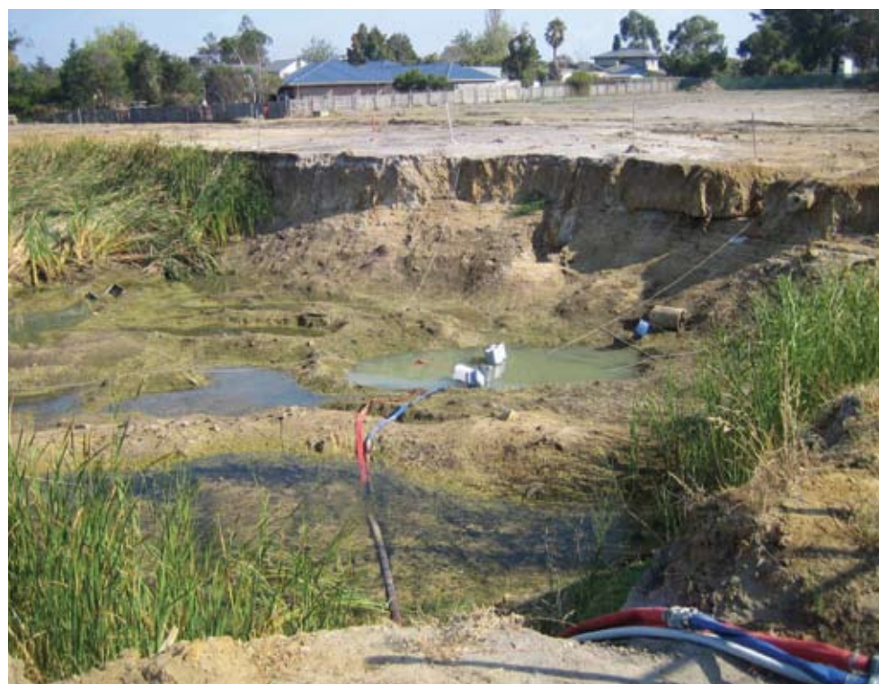
After: More than two million litres of rainwater was extracted and used to water more than 3,000 drought affected street, park and reserve trees. Photo: GLG Developments.
