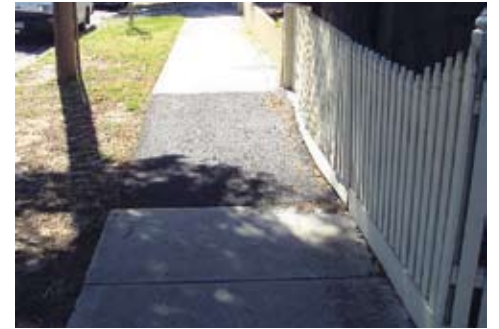
After treatment with asphalt. Photo: GlenWorks.
