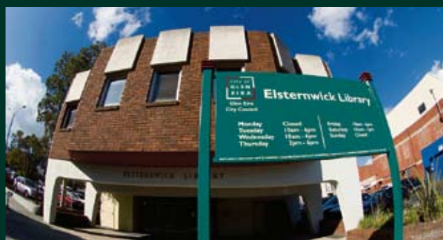
$100,000 will be spent on replacing the ceiling at Elsternwick Library. Photo: Bernie Bickerton.
