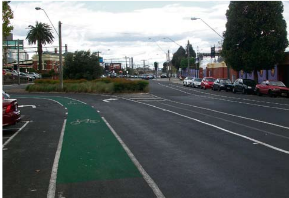
Station Street, Caulfield East. Photo: GECC Traffic Engineering Department.
