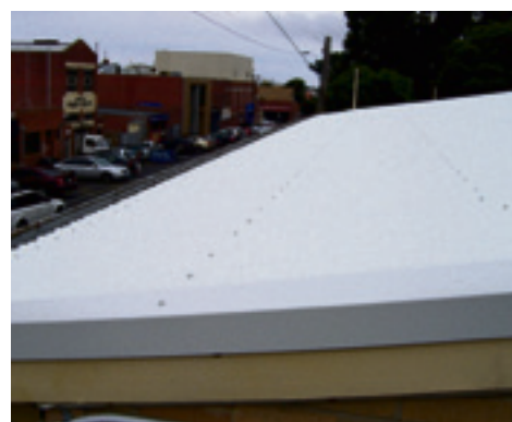
The new roof will help keep the Preschool cool.
