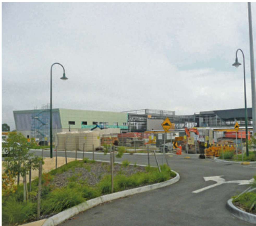
March 2011: GESAC is taking shape. GECC Capital Works.
