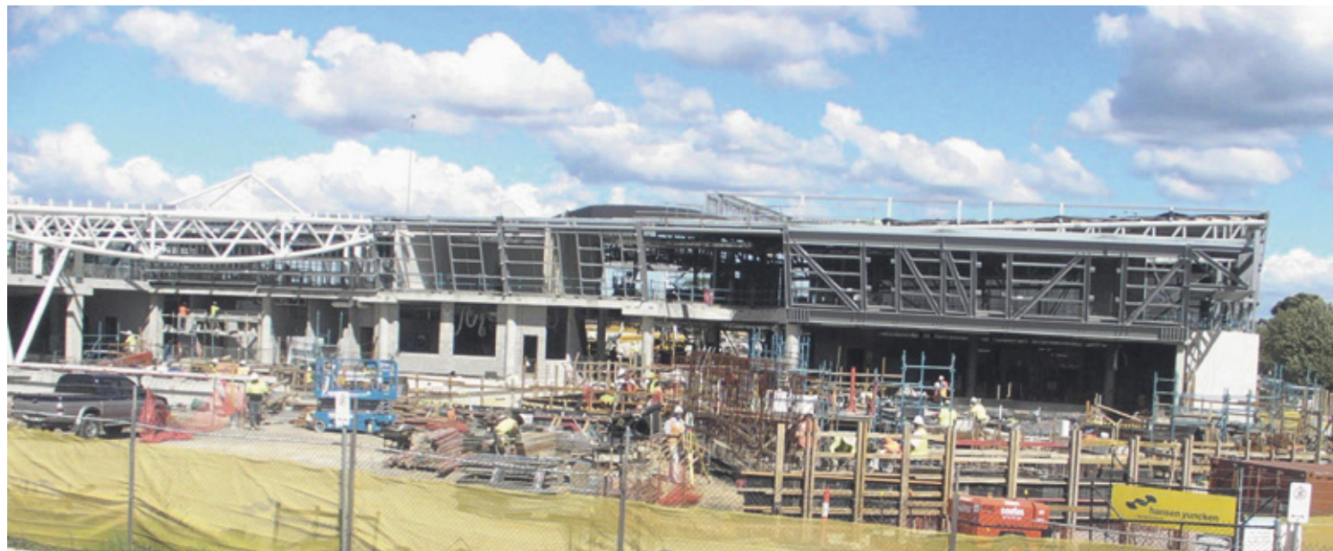
On-site at Glen Eira Sports and Aquatic Centre. Photo: GECC Capital Works.
