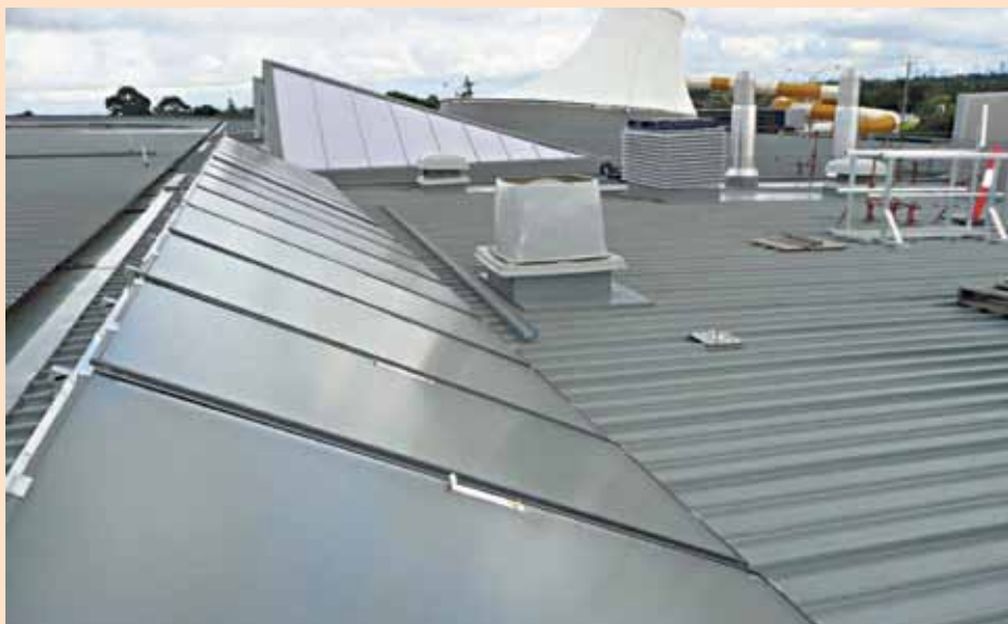
The solar panels will provide hot water for showers and basins. Photo: GECC Capital Works.
