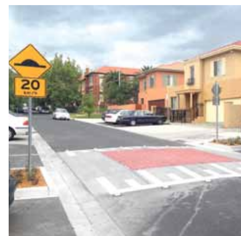
Olive Street, Caulfield South.
