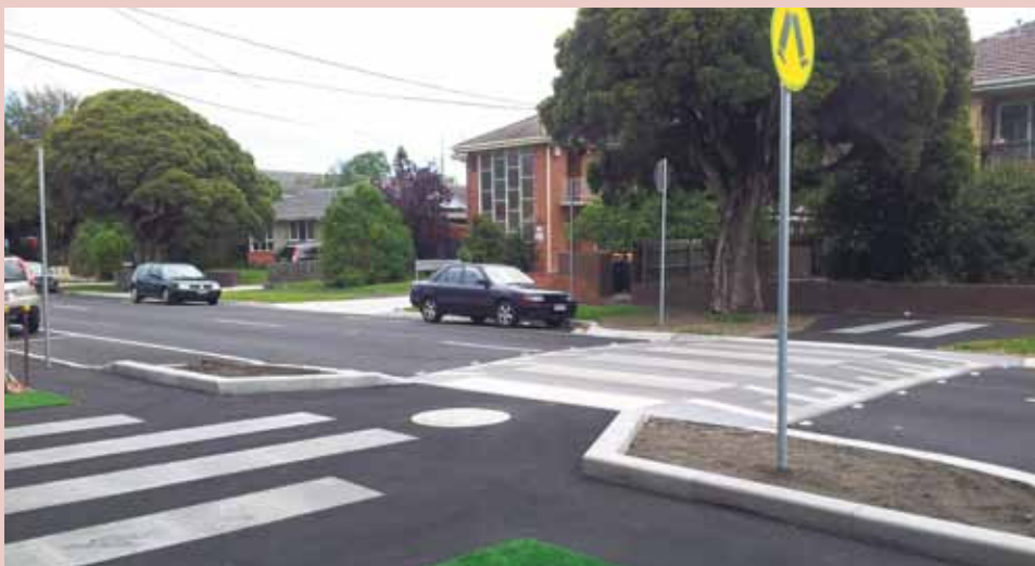
Relocation of road space at Kokaribb Road, Carnegie. Photo: Glen Eira City Council Transport Planning Department.
