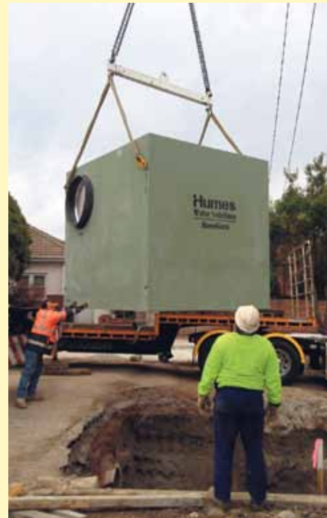
Council's newly installed GPT traps rubbish washed into Council drains from Carnegie Shopping Centre.
