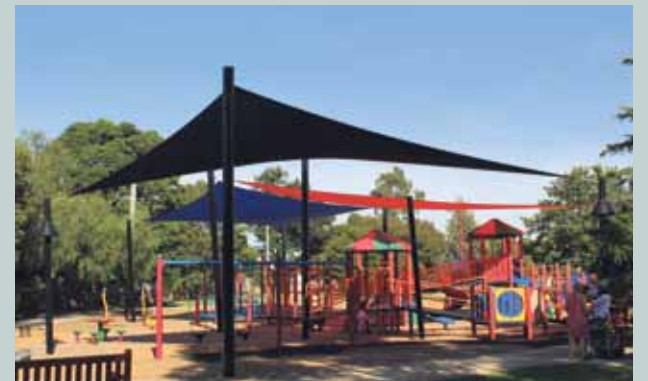
Council has been proactive in installing shade sails and providing shade at numerous playgrounds throughout Glen Eira.
