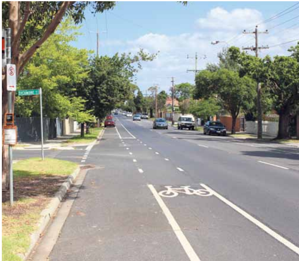
Council has added bicycle lanes to Booran Road, Tucker Road and Koornang Road to promote and encourage cycling.
