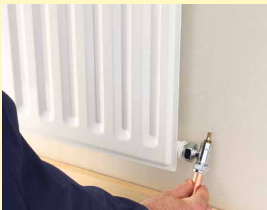
It is recommended that all heaters be professionally installed and that they are serviced every two years.
